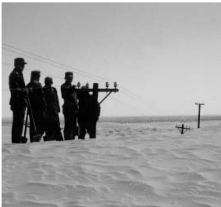
After sand storms, electricity and telephone poles are often buried in the drifting sand dunes. In order to keep systems working, soldiers have to raise the lines by extending the pole. Photo: Lu Tongjing.
